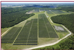
To date, Kimley-Horn has completed more than 600 solar development projects across the US.
